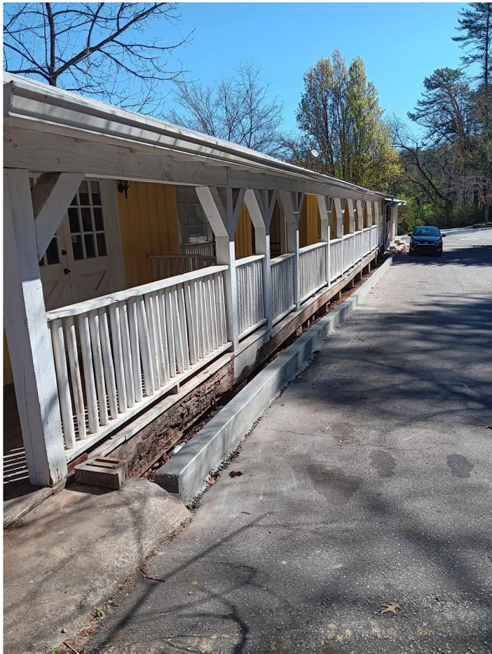
PROGRESS ON DIVERTING THE RUNOFF that was undermining the support piers under the Fellowship Hall. Bates Concrete has trimmed the asphalt and poured the concrete barrier along Heritage Hollow Drive, now that we have been blessed with warmer temperatures. Removing the old lattice has revealed more problems to be addressed, but we are making headway on this project.
